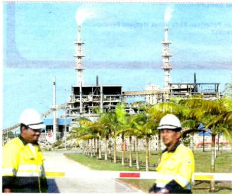
The entrance to the Lynas plant in Gebeng, Kuantan.
